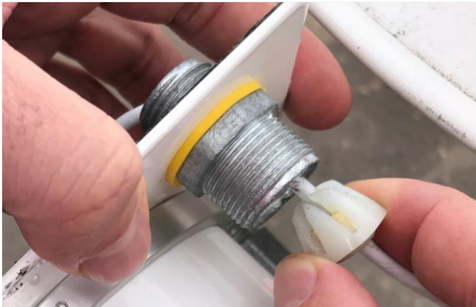
Figure 14. Remove White Cable Clamp
