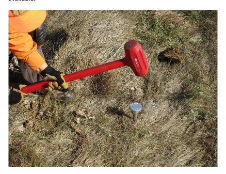
Figure 30. Use a sledgehammer to seat the cap and drive the rod to the desired position
