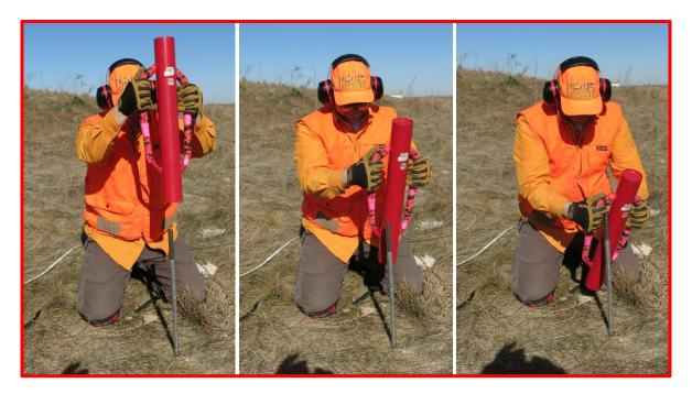
**Figure 29.** Do not lift the post diver above the top of the rod during the striking motion as the worker could injure their leg or hand
