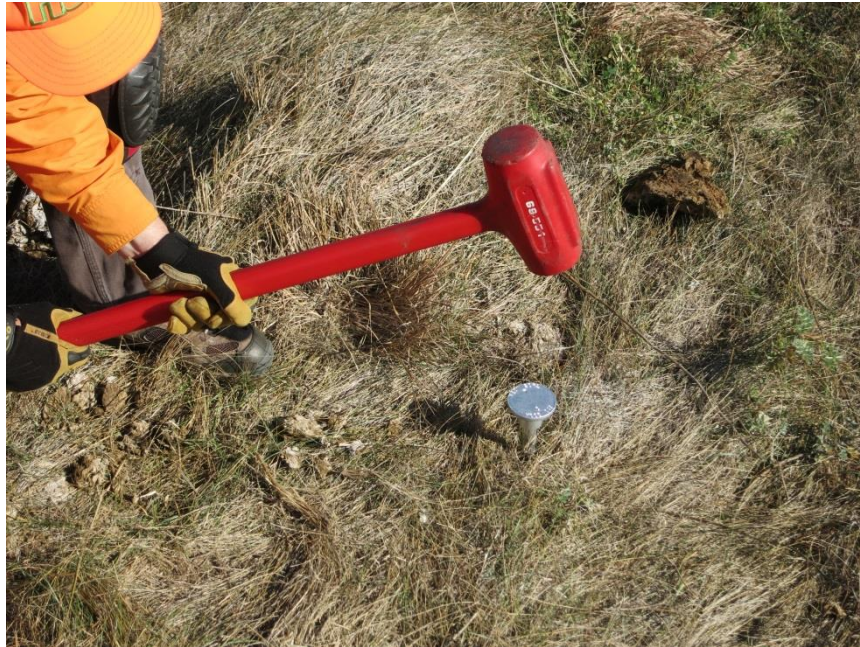
Figure 16. Use a sledgehammer to seat the cap and drive the rod to the desired position.
