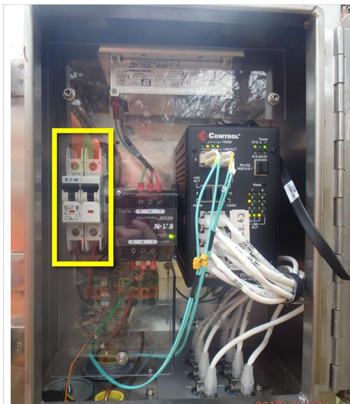
Figure 137. AIS Combination Box - 5 Amp Breakers
