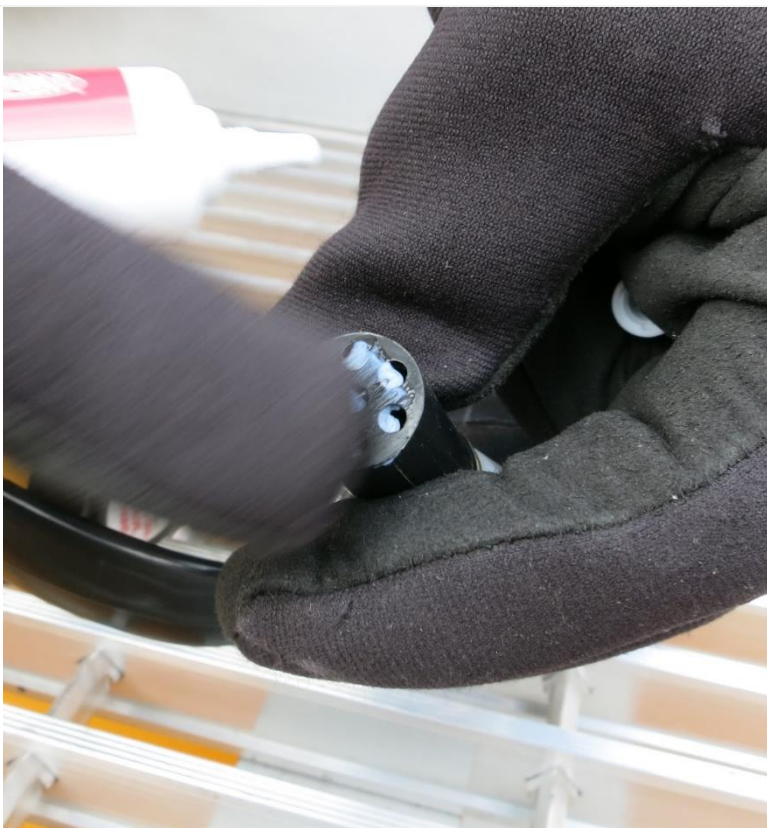
Figure 27. Apply Krytox to Female 6-Pin Connectors
