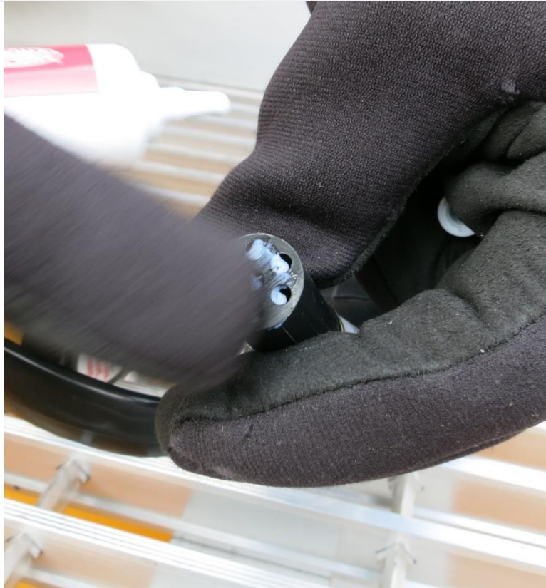
Figure 27. Apply Krytox to Female 6-Pin Connectors
