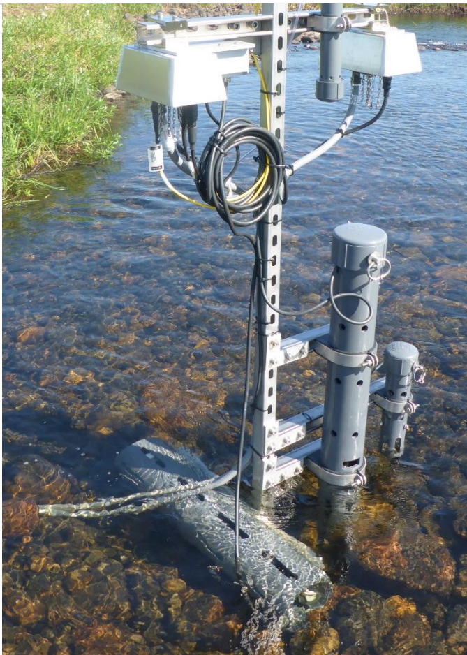
Figure 132. Multisonde Cable Dressing - Complete Installation
