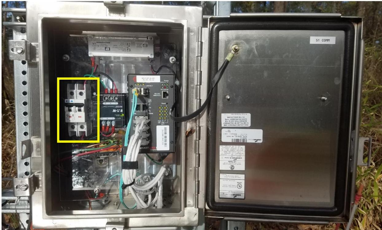
Figure 18. Flip circuit breakers down to turn off power (This combo cox is live - Power is ON)
