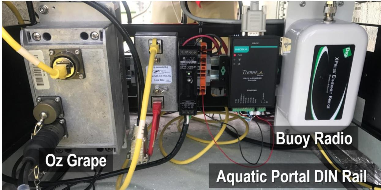
Figure 17. Aquatic portal precip DIN rail: AIS buoy portal radio/Oz grape subsystem
