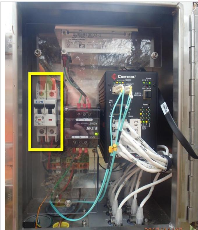
**Figure 121. AIS combination box - 5 amp breakers**
