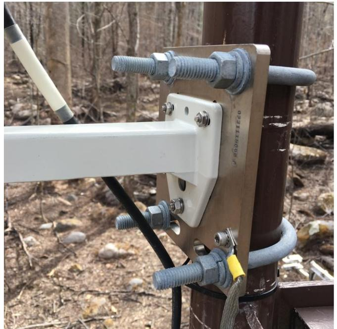
**Figure 13.** Camera U-bolts and Grounding Cable on TIS Tower Leg.
