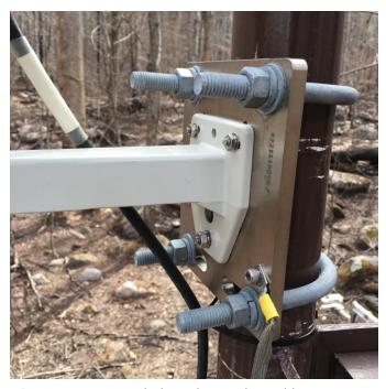
**Figure 13**. Camera U-bolts and Grounding Cable on TIS Tower Leg.
