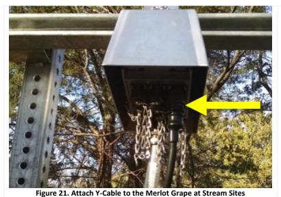
**STEP 6.1** | <u>Stream sites:</u> Attach the Y cable to the 12V Merlot Grape in the same 12-10 connector as the sensor power cable (Figure 21).
