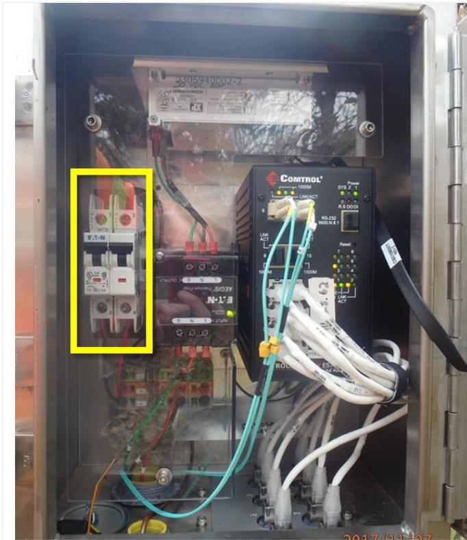
**Figure 68. AIS Combination Box - 5 Amp Breakers**
