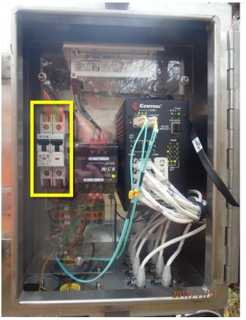
Figure 71. AIS Combination Box - 5 Amp Breakers
