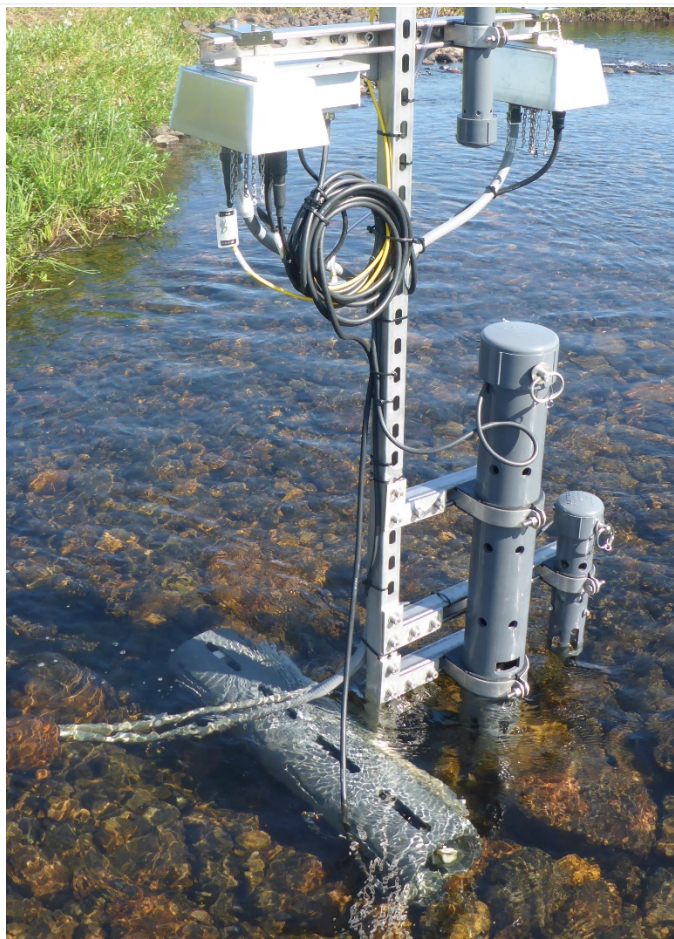
Figure 68. SUNA cable dressing
