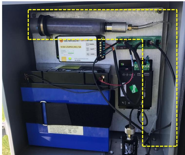
**Figure 20. Desiccant Location in GWW Radio/Power Box (D09)**
