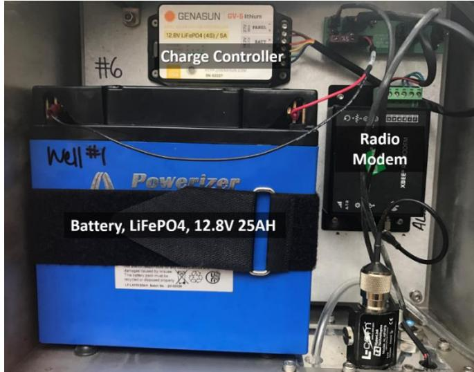
Figure 4. Power/Telemetry Components in GWW NEMA Enclosure
