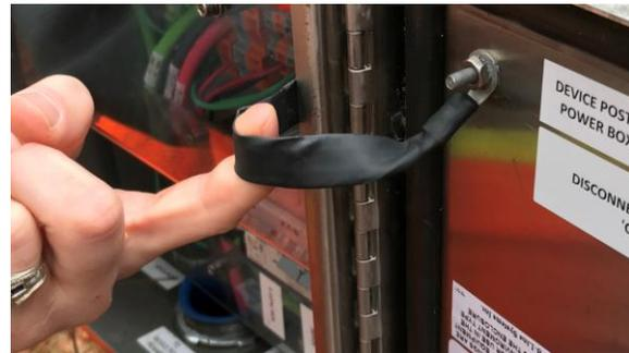
**Figure 10. Combo Box Ground Strap**
