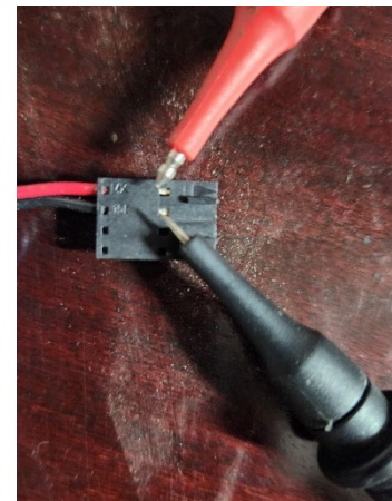
Figure 53. DMM Test on Non-In-Situ External Battery
