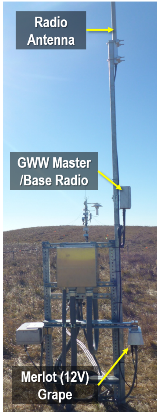
Figure 4. GWW DAS Components on Aquatic Met Station Device Post
