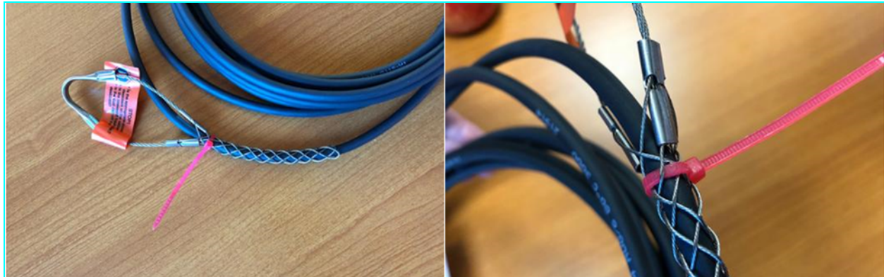
Figure 25. Secure Mesh Wire Basket to Sensor Cable
