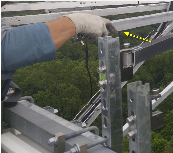
Figure 64. Move Crossbeam Toward Tower Top Railing
