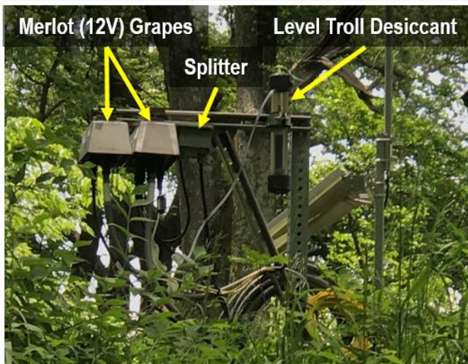
Figure 91. Grape (12V) High-Water Installation (D06 KING)
