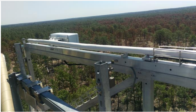
Figure 69. Rotate Assembly Toward Tower Top Railing/Deck
