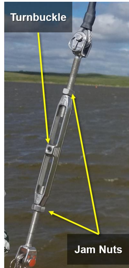
Figure 20. Guy-wire Components
