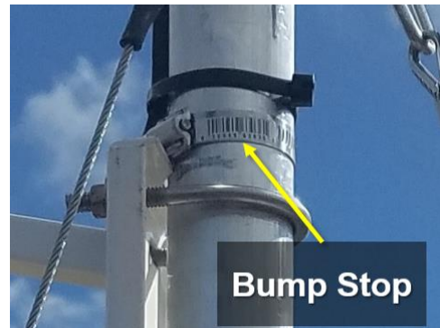
Figure 18. Bump Stop on Met Mast
