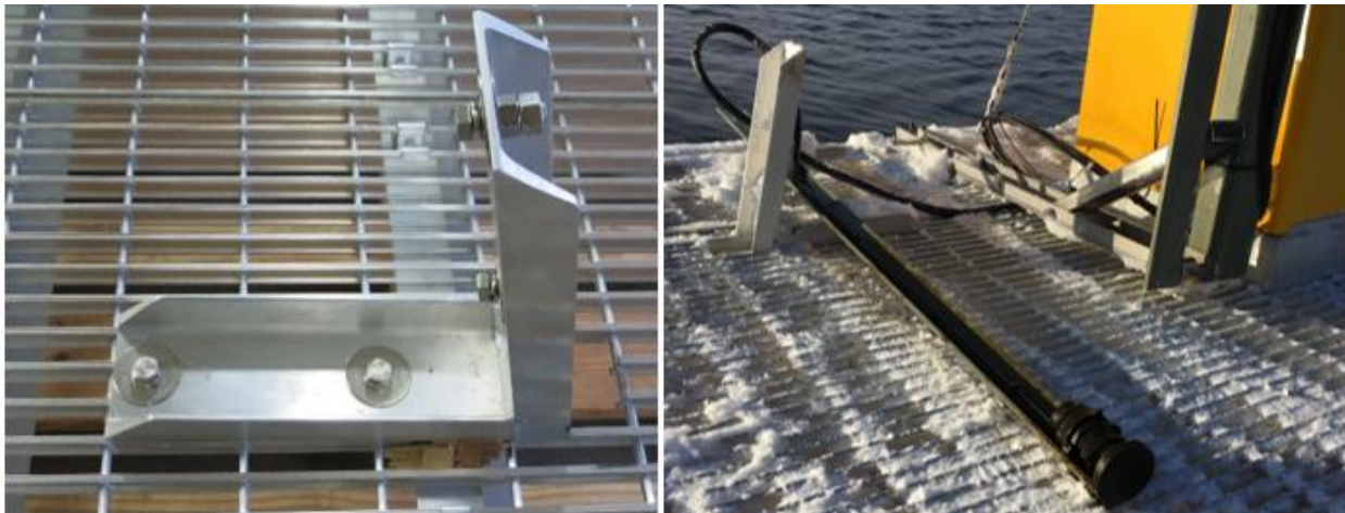
Figure 22. Depth Sounder Bracket (Left) and Depth Sounder Instrument (Right) on Floating Deck
