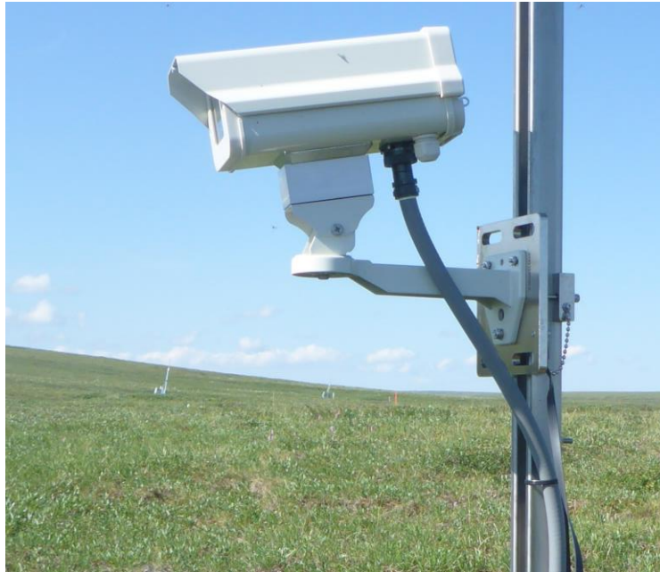
Figure 14. Remove Digital Network Cable from Unistrut at an AIS Site
