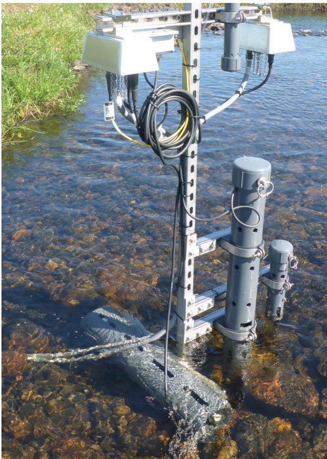
Figure 78. SUNA Cable Dressing - Complete Installation
