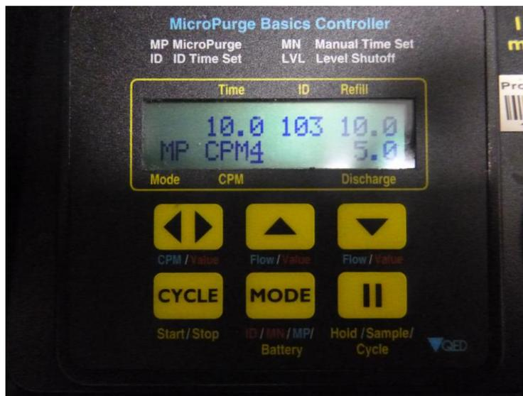
**Figure 20.** Groundwater pump control panel screen. Note the Refill and Discharge times on the right.
