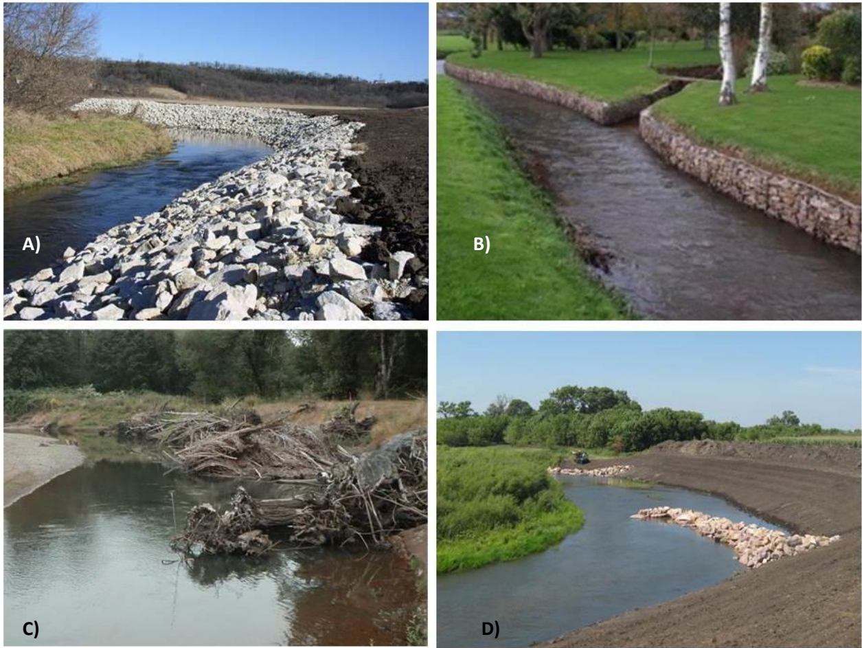
Figure 12. Examples of shoreline revetments a) rip-rap with rock, b) gabion baskets filled with rock, c) soft armoring using root wads and logs, and d) in-stream rock J-hook for modifying flow.
