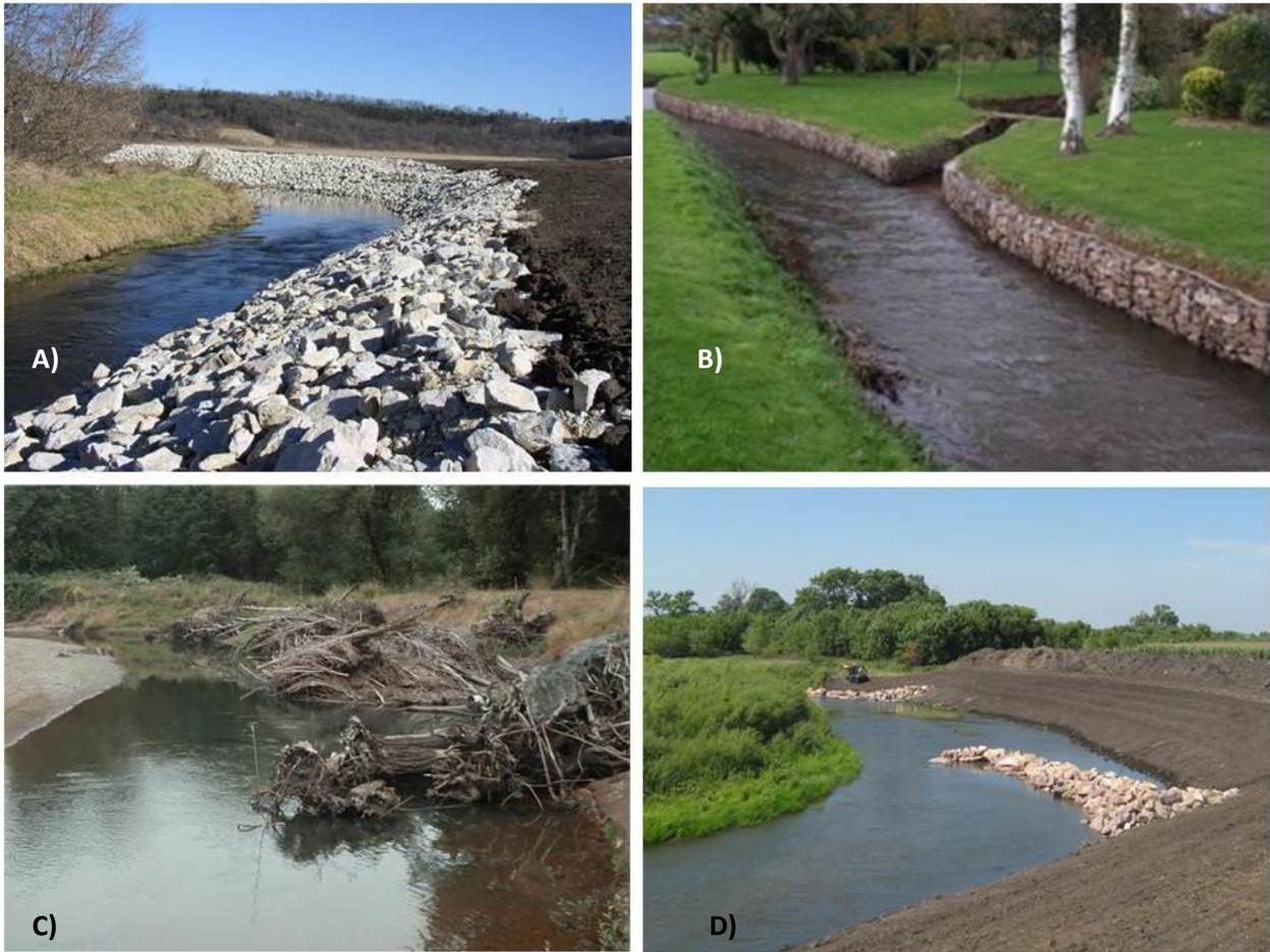
**Figure 6.** Examples of shoreline revetments a) rip-rap with rock, b) gabion baskets filled with rock, c) soft armoring using root wads and logs, and d) in-stream rock J-hook for modifying flow.
