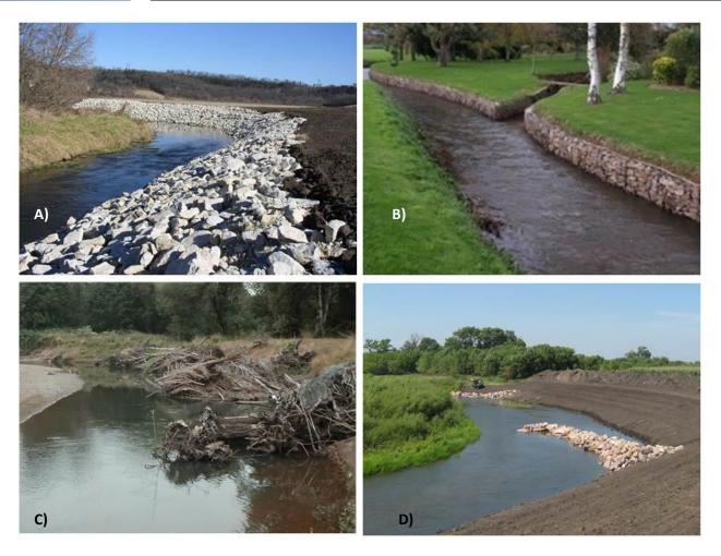
**Figure 6.** Examples of shoreline revetments a) rip-rap with rock, b) gabion baskets filled with rock, c) soft armoring using root wads and logs, and d) in-stream rock J-hook for modifying flow.
