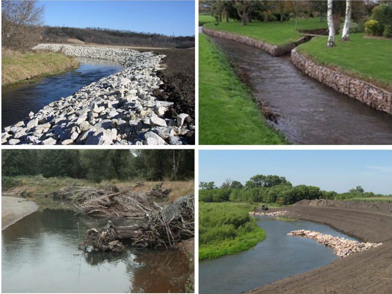
Figure 17. Examples of bank revetments. A) rip-rap with rock; B) gabion baskets filled with rock; C) soft armoring using root wads and logs; D) in-stream rock J-hook for modifying flow.
