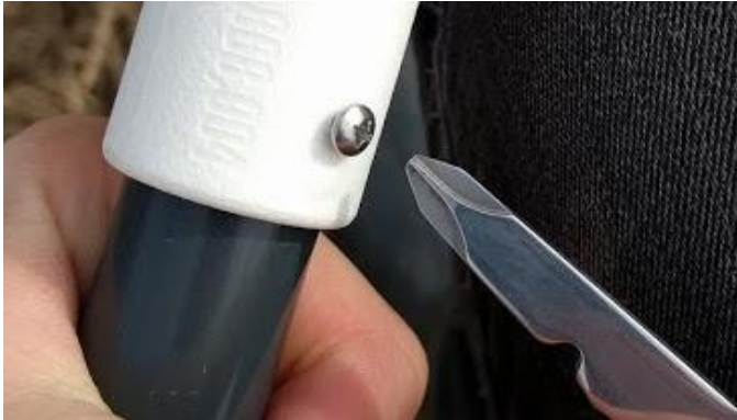
Figure 31. Screw Surge Block to PVC TIGHTLY (D10 ARIK)
