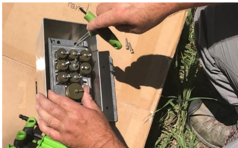
Figure 45. Remove Grape from Grape Shields (D06 KING)
