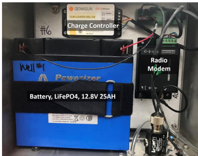
Figure 4. Power/Telemetry Components in GWW NEMA Enclosure
