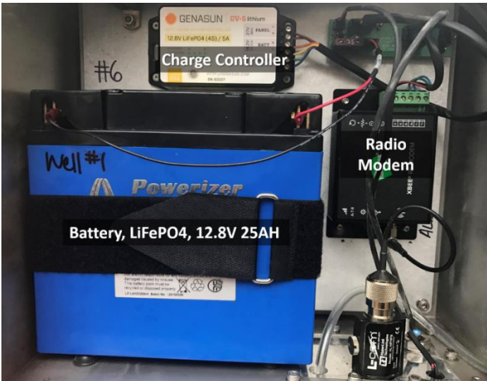
Figure 4. Power/Telemetry Components in GWW NEMA Enclosure
