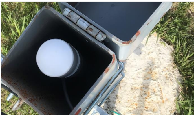
Figure 38. Place Cap on GWW and Secure Cover (D09 PRLA)
