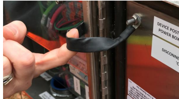
Figure 10. Combo Box Ground Strap
