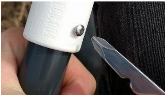
Figure 32. Screw Surge Block to PVC TIGHTLY (D10 ARIK)
