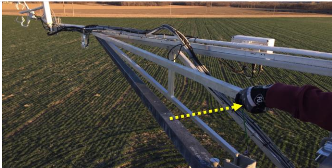
Figure 65. Guide the Boom Arm Toward the Tower Top (D06 KONA)
