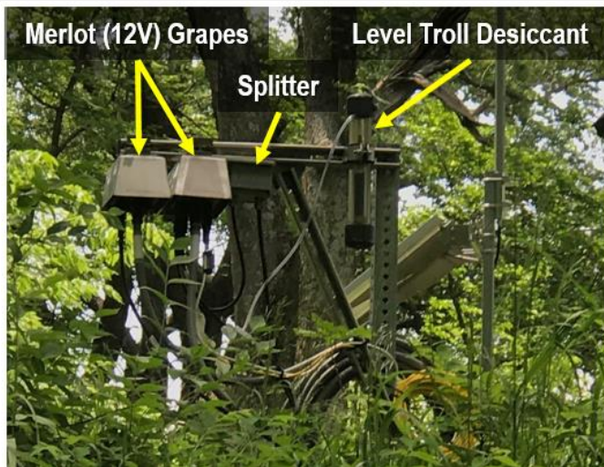
Figure 91. Grape (12V) High-Water Installation (D06 KING)
