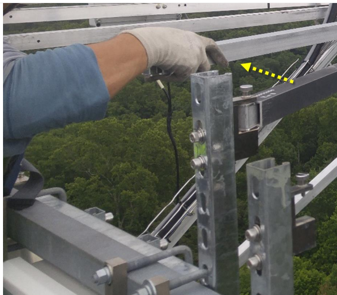
Figure 64. Move Crossbeam Toward Tower Top Railing
