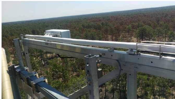
Figure 69. Rotate Assembly Toward Tower Top Railing/Deck
