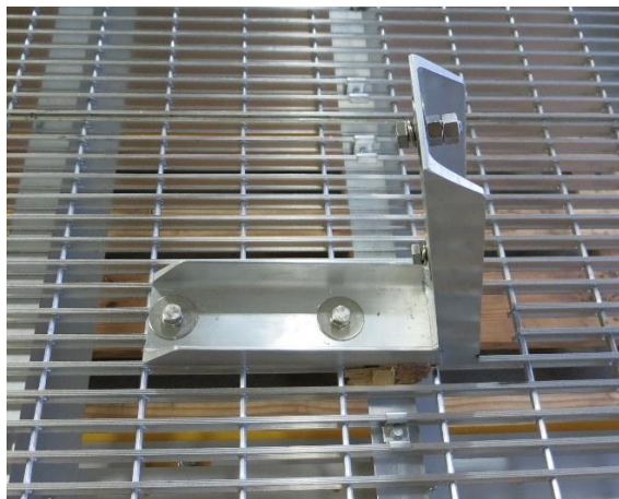
Figure 18. Depth Sounder Bracket on Floating Deck
