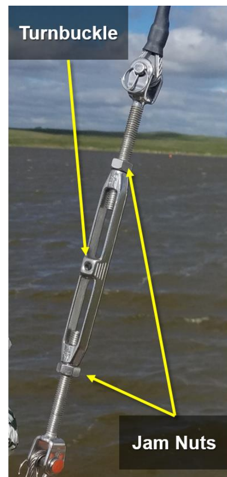
Figure 20. Guy-wire Components
