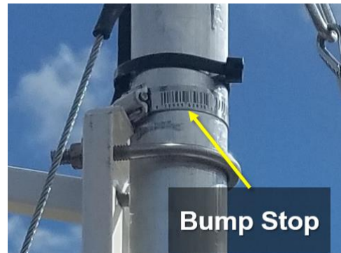
Figure 18. Bump Stop on Met Mast
