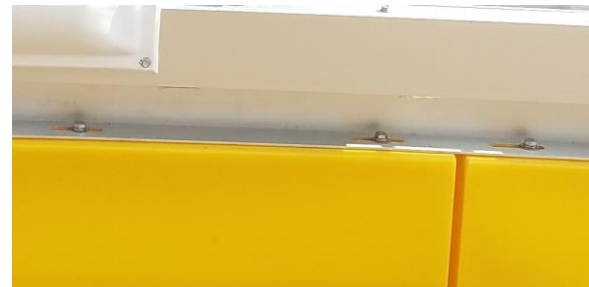
Figure 9. Attachment Points for Floating Deck & Pontoon
