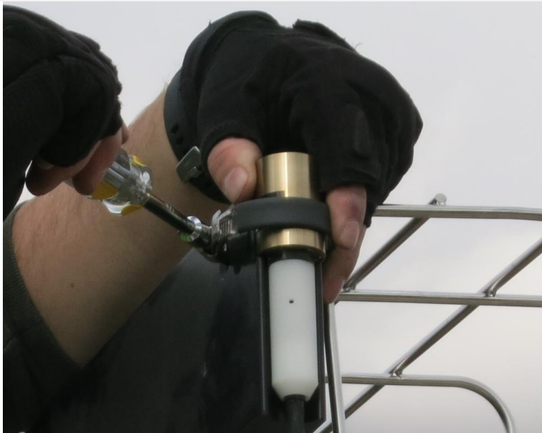
Figure 65. Secure Sensor in Mount
