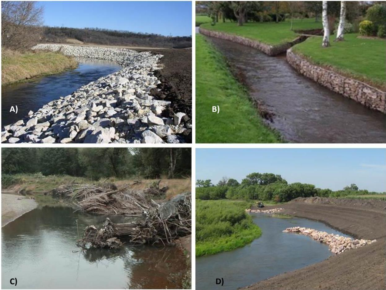
**Figure 9.** Examples of shoreline revetments a) rip-rap with rock, b) gabion baskets filled with rock, c) soft armoring using root wads and logs, and d) in-stream rock J-hook for modifying flow.
