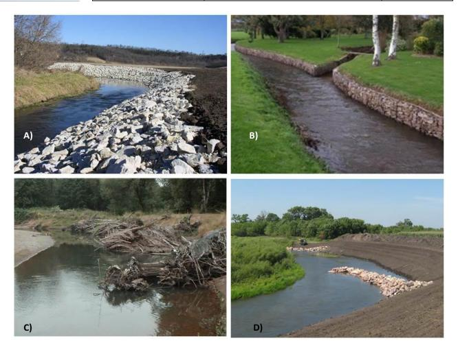
**Figure 9.** Examples of shoreline revetments a) rip-rap with rock, b) gabion baskets filled with rock, c) soft armoring using root wads and logs, and d) in-stream rock J-hook for modifying flow.
