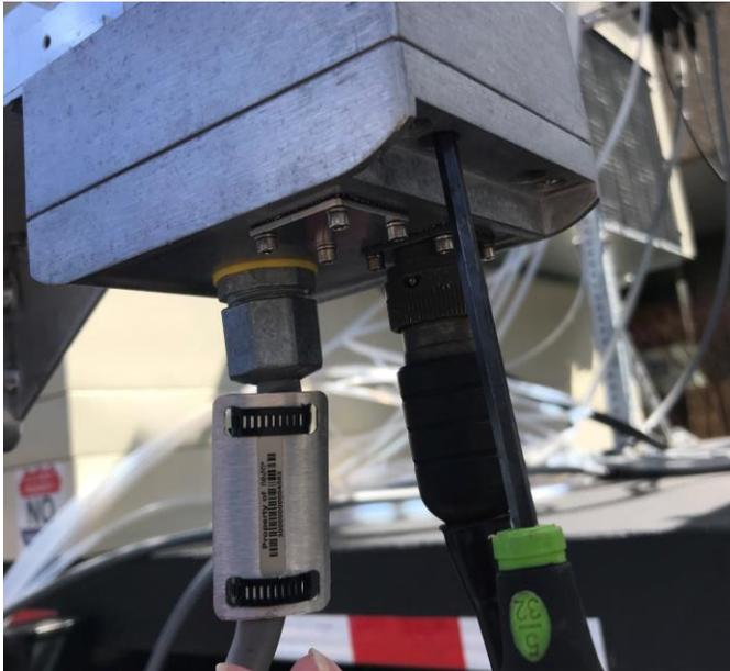
Figure 21. Remove Junction Box from Boom (NEON HQ).
