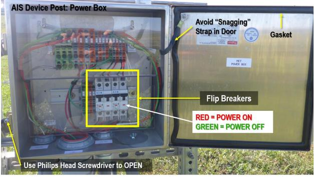
Figure 34. AIS Device Post: Power Box Components (Domain 18 OKSR AIS Aquatic Met Station).
