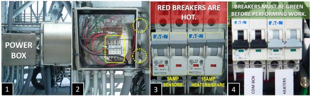
Figure 33. How to Power Down a Tower ML.
