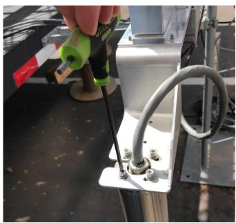
Figure 19. Remove 2D Wind Sensor (NEON HQ).
