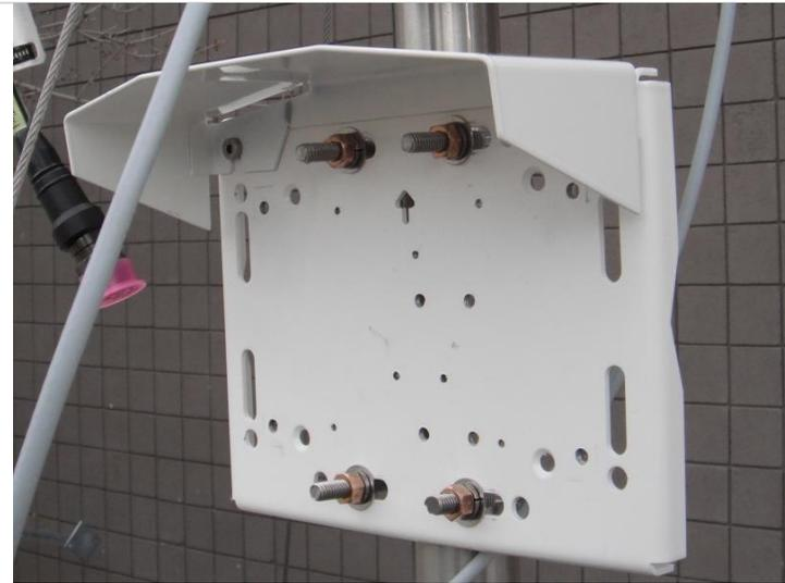
Figure 15. Pole Mount Plate with U-bolts (Source: RD [08]).
