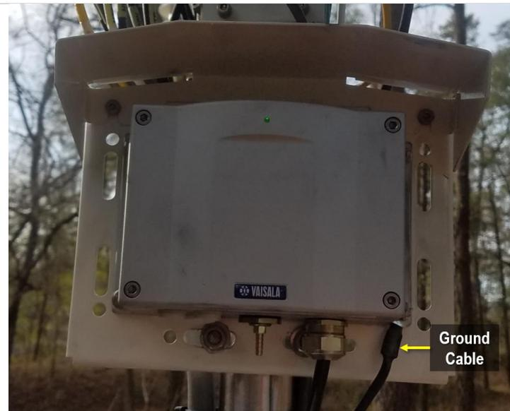
Figure 16. Install Sensor onto Mount Plate (Source: D03 FLNT).
