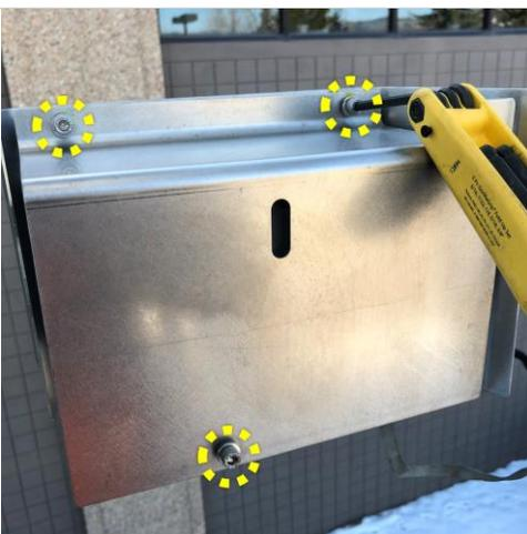
**Step 4.** (TIS Only) Using a  $\frac{3}{16}$ " Allen key, loosen the three screws holding on the front sun shield.
