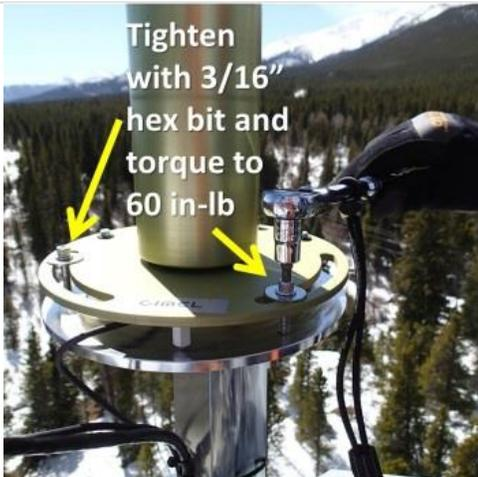
**Step 5.** Once aligned, tighten down the three socket head screws with a 3/16" hex bit, and torque to 60 in-lb.
