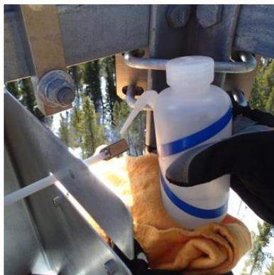
**Step 7.** Visually inspect the wet sensor for caked on dirt, or bird droppings.
