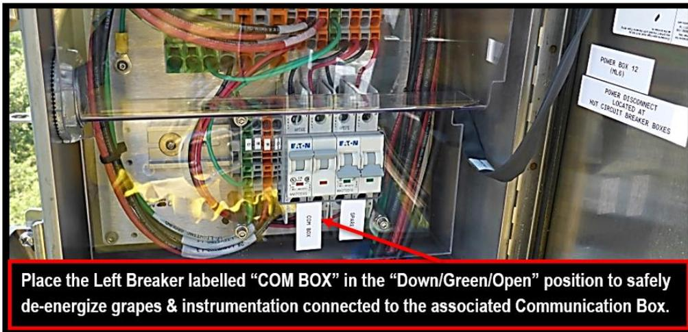
**Figure 24.** De-energize the GRAPE before disconnecting the sensor cables.
