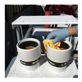
**Step 3.** Clean both white chimney caps by wiping down the neck of the chimneys. Start from the top of the chimney down. Re-apply cleaner to the lint-free cloth, if necessary.
