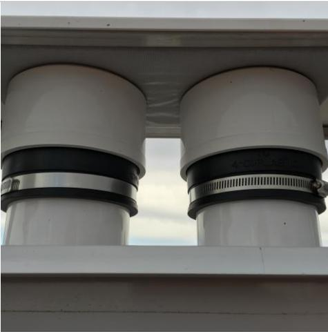
**Step 4.** Inspect the seal between the bottom of the Moving Cover and the top of the two chimneys.
