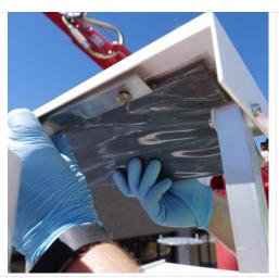
**Step 7.** Smooth out the new lid seal and slide it under the aluminum bar that was loosened in **Step 3** above.
