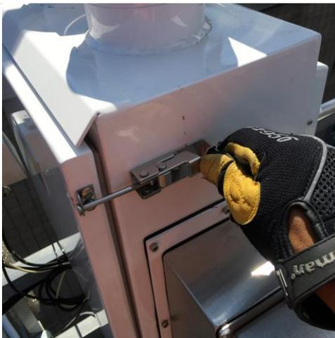
**Step 3.** Close and secure the door to the collector.
