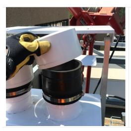
**Step 7.** Replace the PVC cap on each chimney.
