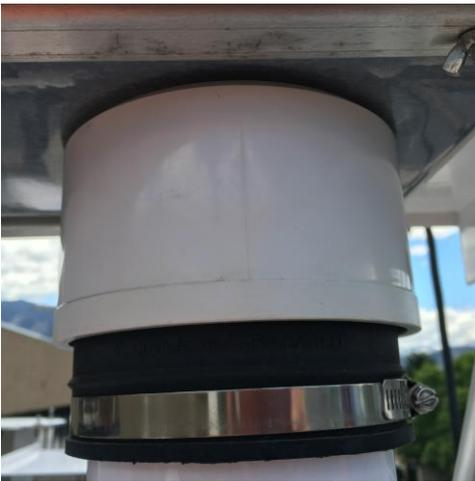
**Step 5.** Inspect the black rubber gasket and the hose clamp.
