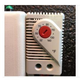
**Step 1.** Verify the set point is ~37 °F via the Temperature Controller on top of the power supply (see **Figure 5**).
