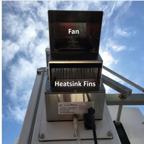
**Step 1.** Look underneath the shroud of the thermo-electric chiller unit. Inspect the fan and heatsink fins.
