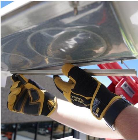
**Step 4.** Loosen and remove the wing nuts on the other side along with the aluminum bar.
