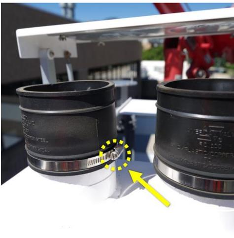
**Step 6.** Once adjusted to the appropriate height, tighten the hose clamps.
