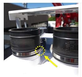
**Step 6.** Once adjusted to the appropriate height, tighten the hose clamps.
