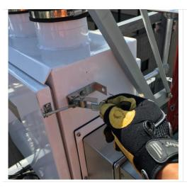
**Step 3.** Unlatch the two latches on the closed door and open the door.
