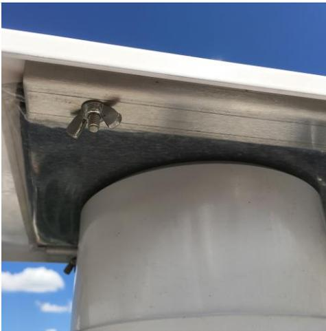
**Step 13.** Check the seal between the Moving Cover and the top of the chimneys once more.
