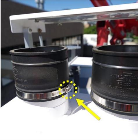
**Step 4.** Loosen the hose clamp enough to the rubber gasket up and down.
