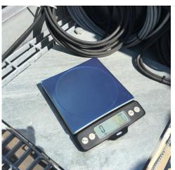
Step28. Remove the field scale from its travel case and turn on. Place in a stable, flat and level location and zero the scale.
