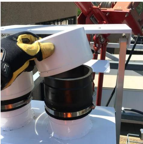
**Step 3.** Remove the PVC cap from each chimney.
