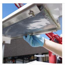
**Step 9.** Hold the aluminum bar in place and hand tighten on the wing nuts.
