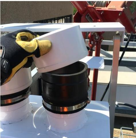
**Step 4.** Remove the PVC cap and inspect the gasket. Clean if necessary.
