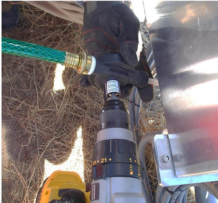
Figure 13. Drill attached to drill pump.
