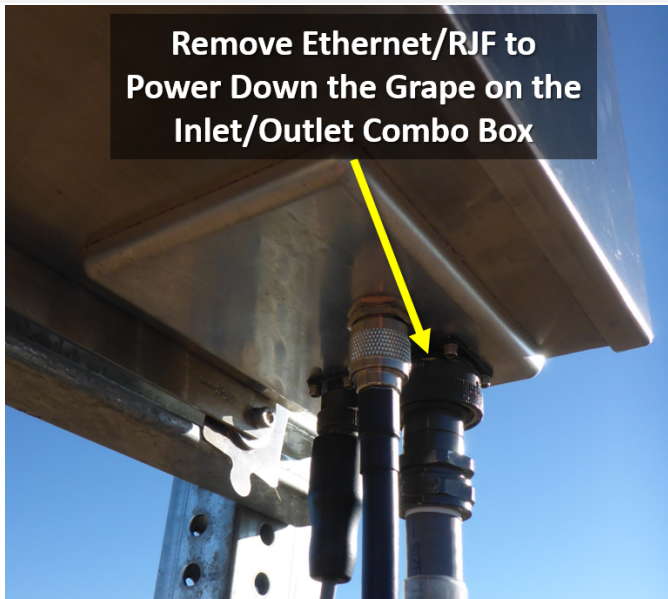
Figure 12. Power Down Site from Combo Box
