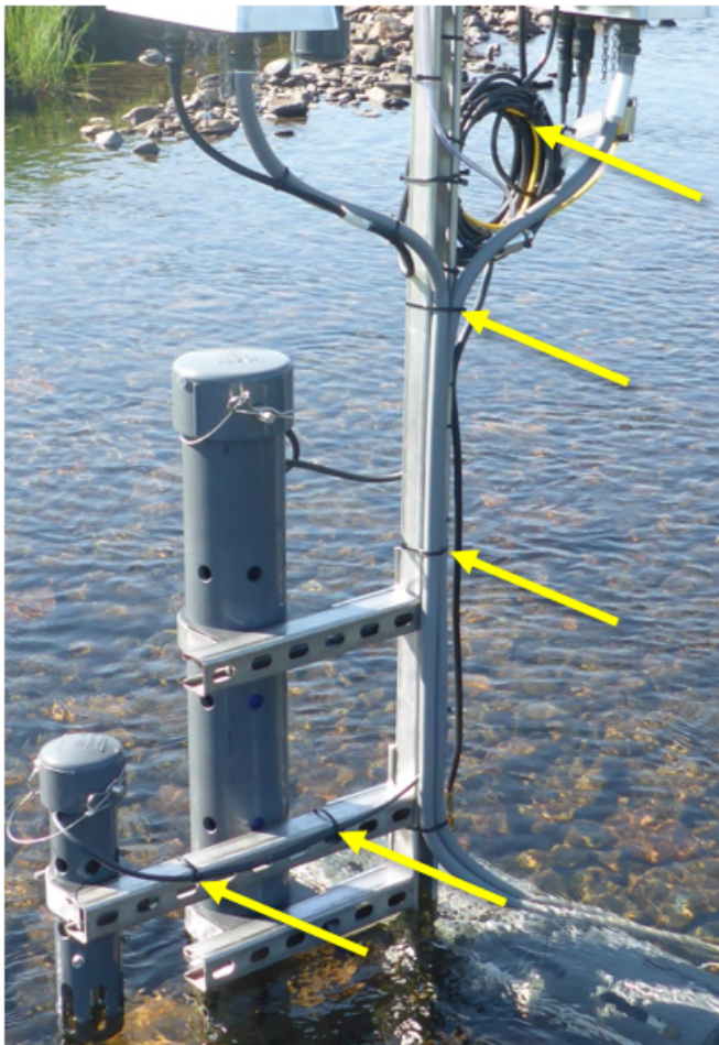
Figure 23. Secure Cables using Zip Ties (D18 OKSR)
