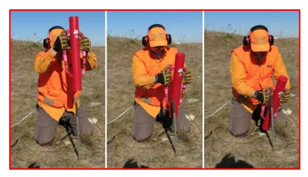
Figure 13. Do not lift the post diver above the top of the rod during the striking motion as the worker could injure their leg or hand
