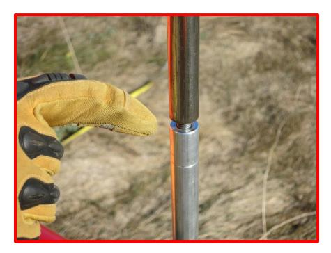
Figure 12. Do not allow the monument assembly sections to become separated while striking
