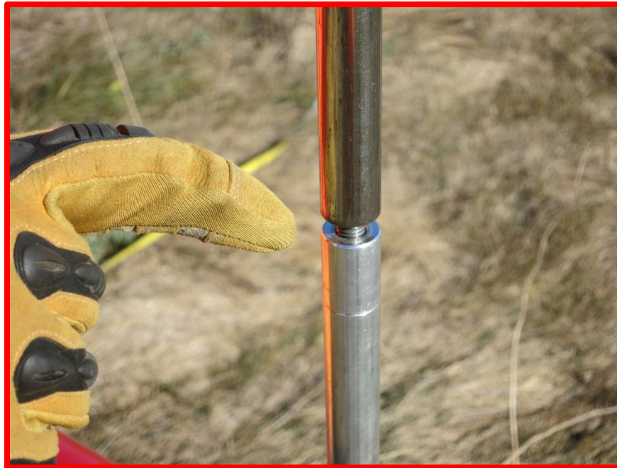
Figure 18. Do not allow the monument assembly sections to become separated while striking
