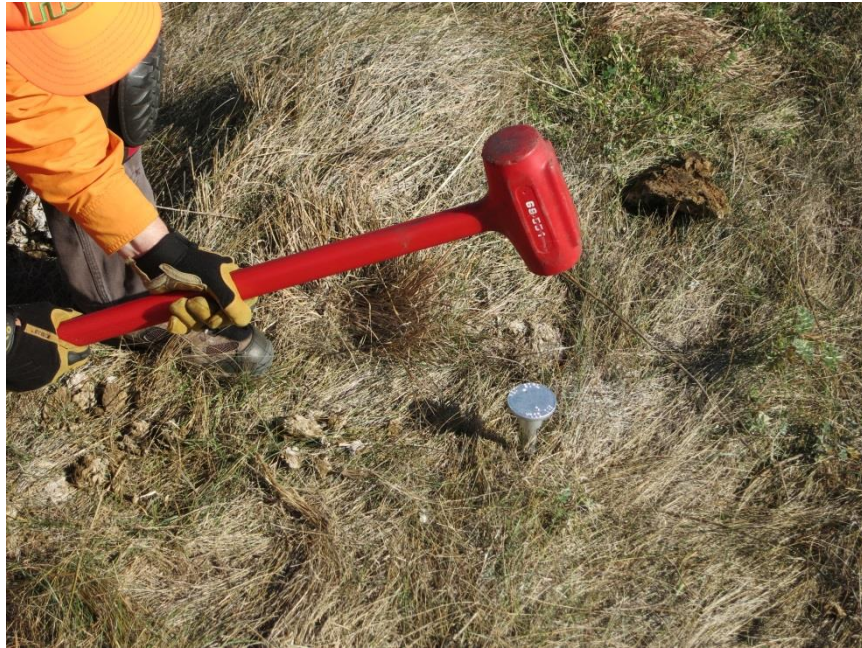
Figure 20. Use a sledgehammer to seat the cap and drive the rod to the desired position
