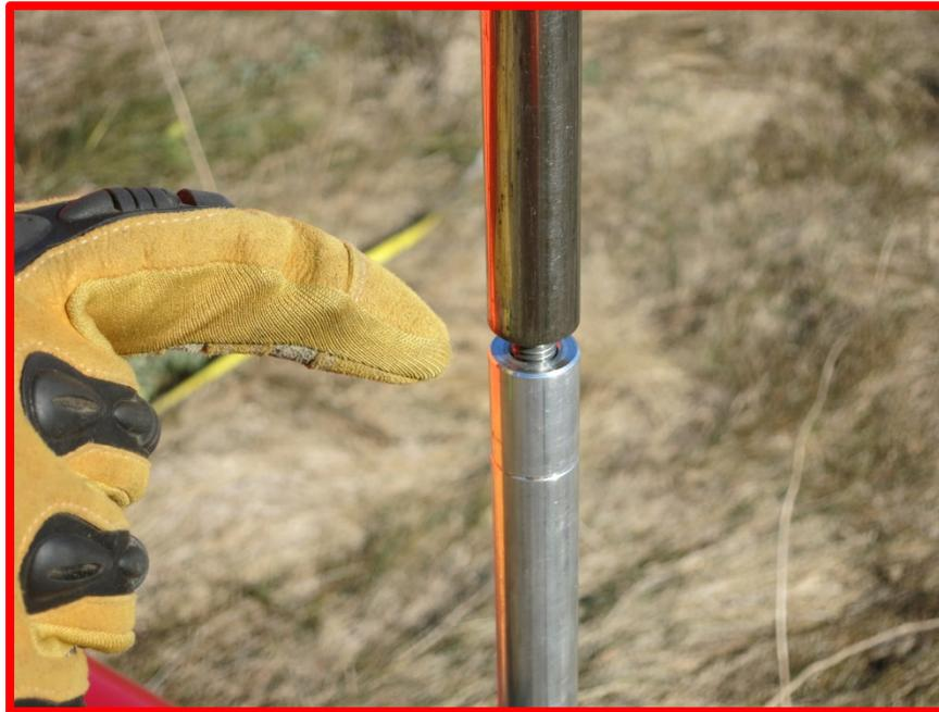
**Figure 28.** Do not allow the monument assembly sections to become separated while striking
