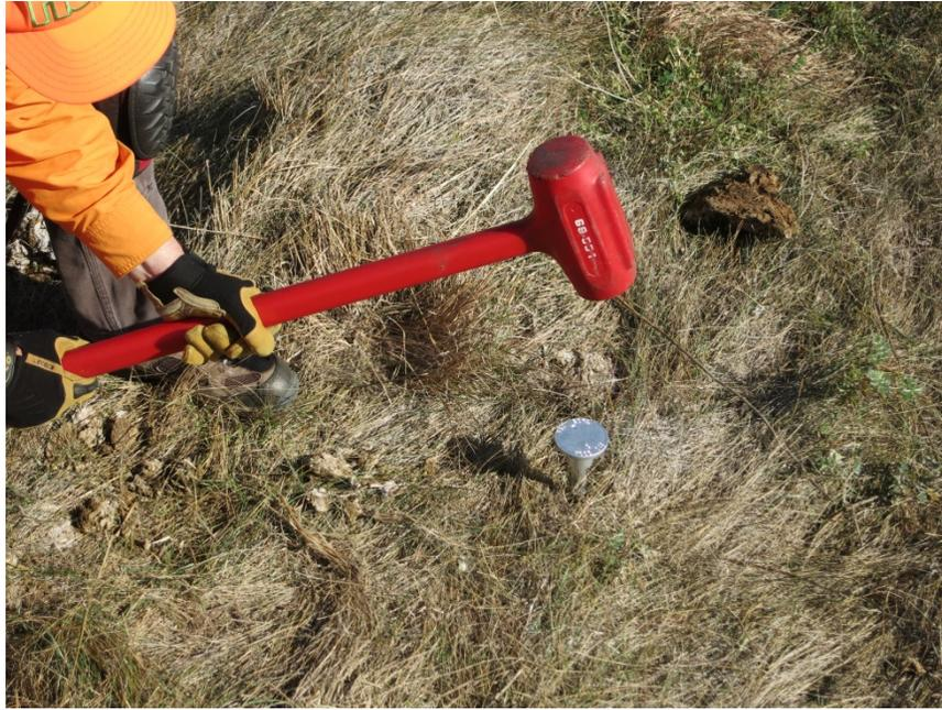
**Figure 30.** Use a sledgehammer to seat the cap and drive the rod to the desired position
