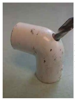
Drill а hole in the back of each 90 degree elbow, as shown.
