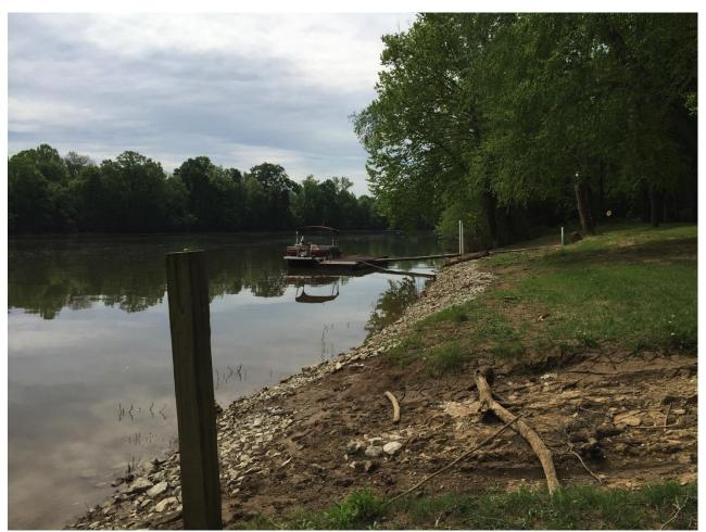
Figure 44. The substrate it mostly sand and silt. Rock and riprap have been added by private land owners to limit bank erosion.
