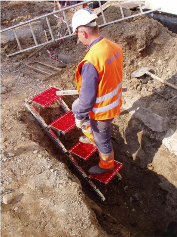
**Figure 17** Picture of installed narrow section of Tuff Steps.
