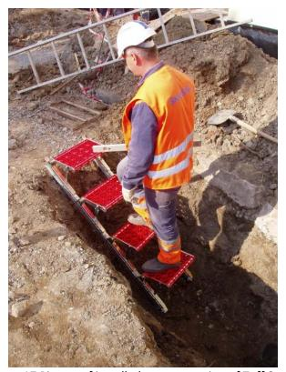
Figure 17 Picture of installed narrow section of Tuff Steps.
