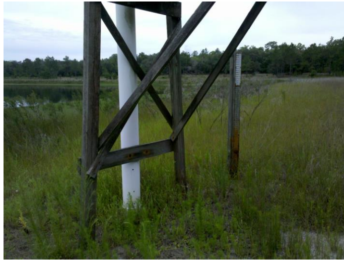
Figure 9 The existing pier in D03 Lake Barco with old staff gauge. The water levels are low and the end of the pier is not submerged.
