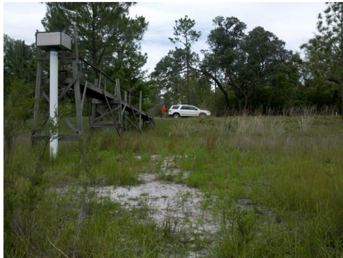
Figure 10 Current access location in D03 Lake Barco and the existing pier.
