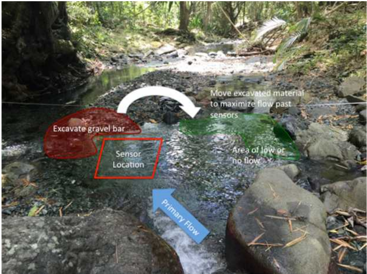
Figure 11. Downstream perspective of S1 location at D04 Río Cupeyes showing the sensor location within the pool (red box), the primary flow (blue arrow), area of excavation (red) within the existing gravel bar and where excavated material is to be delivered (green).
