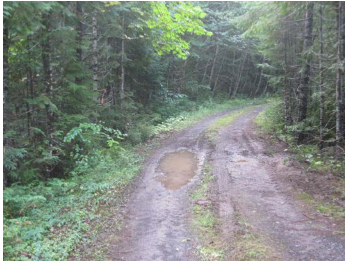
Figure 40 The access road (325) to McRae Creek STREON is well-maintained enough for 2-wheel drive vehicles, except during hazardous winter conditions.
