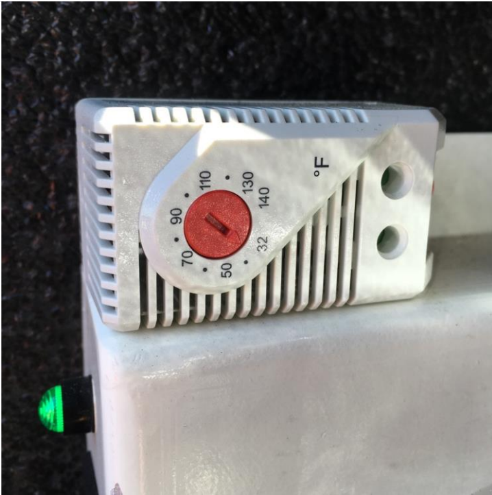
Figure 8. A view of one of the internal Temperature Controllers. See Figure 5 for the location of this Temperature Controller.
