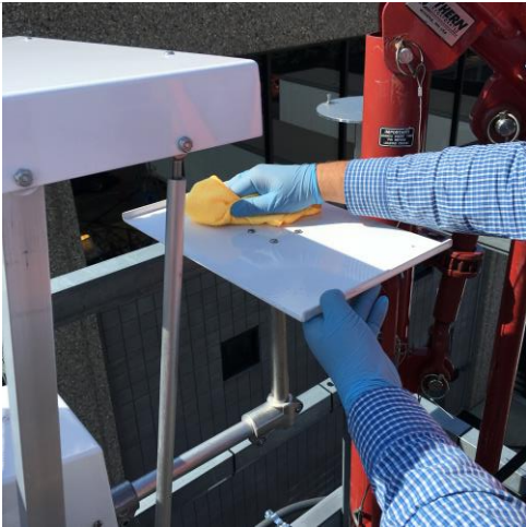
Step 7. Clean the top surface of the Splash Shield.
